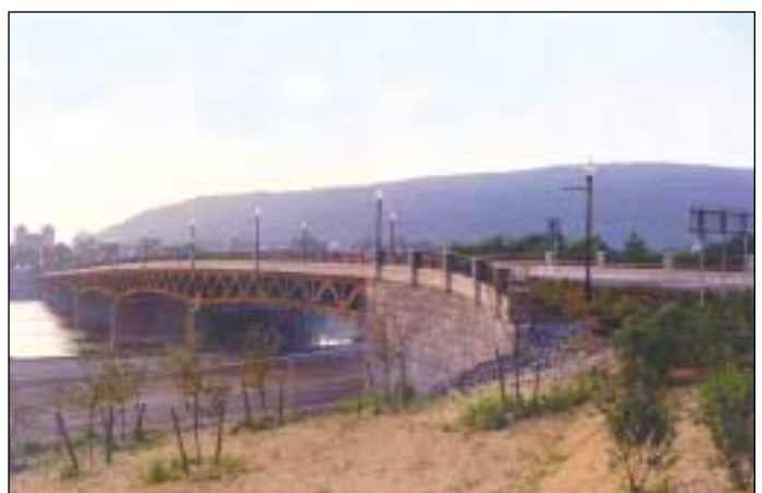
The Court Street Bridge replacement, located in Owego, NY, was a winner of the state's 2004 CSS Exemplary Project Award.
