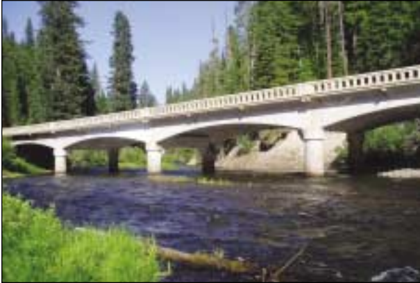
To the left: Located in the Rogue River National Forest, the Rogue River Bridge is one of more than 300 bridges being repaired or replaced in a context-sensitive manner under Oregon’s progressive OTIA III State Bridge Delivery Program.
